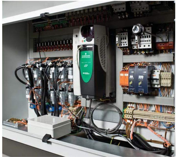
modes – open and closed loop, vector, servo and regenerating modes - connectivity to most industry standard networks and accepting most position feedback protocols. "The Unidrive SP is a very flexible drive," says Direct-Industrial.com managing director John Lenehan. "It proved ideal for this application because of its instant compatibility with the PLC and for its dynamic and accurate response to commands."
