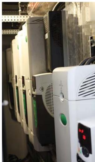
drives, an auxiliary hoisting motor is controlled by a 55kW Unidrive SP AC drive and a travel motor by a 44kW Commander SK AC drive.
