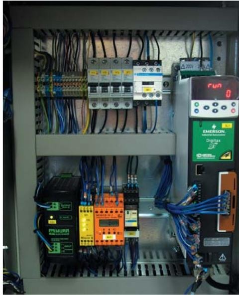
PLC. The system incorporates three feedback loops; a closed position loop, a closed speed control loop and an actual speed control loop using the additional security counter.
