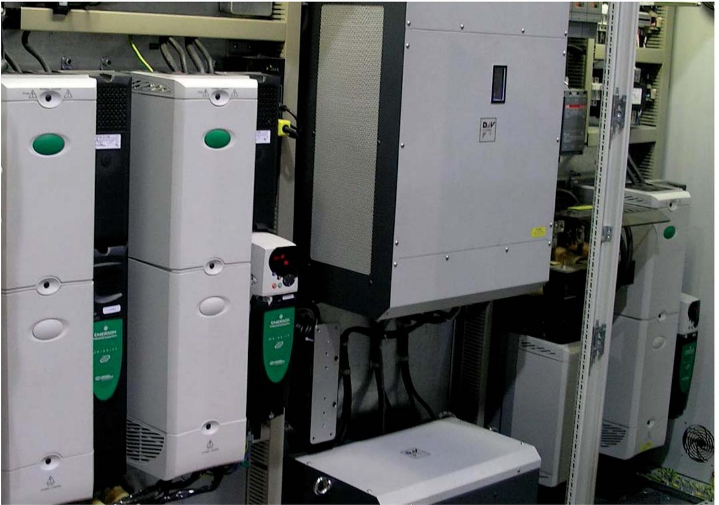
common DC bus. This energy is then available to the tested motor and to other test rigs being run off the same bus. In cases where the tested motor and load motor are operated from differing bus voltages, D&V Electronics developed a unique bidirectional DC-DC converter to allow energy sharing across this multi-level bus.
