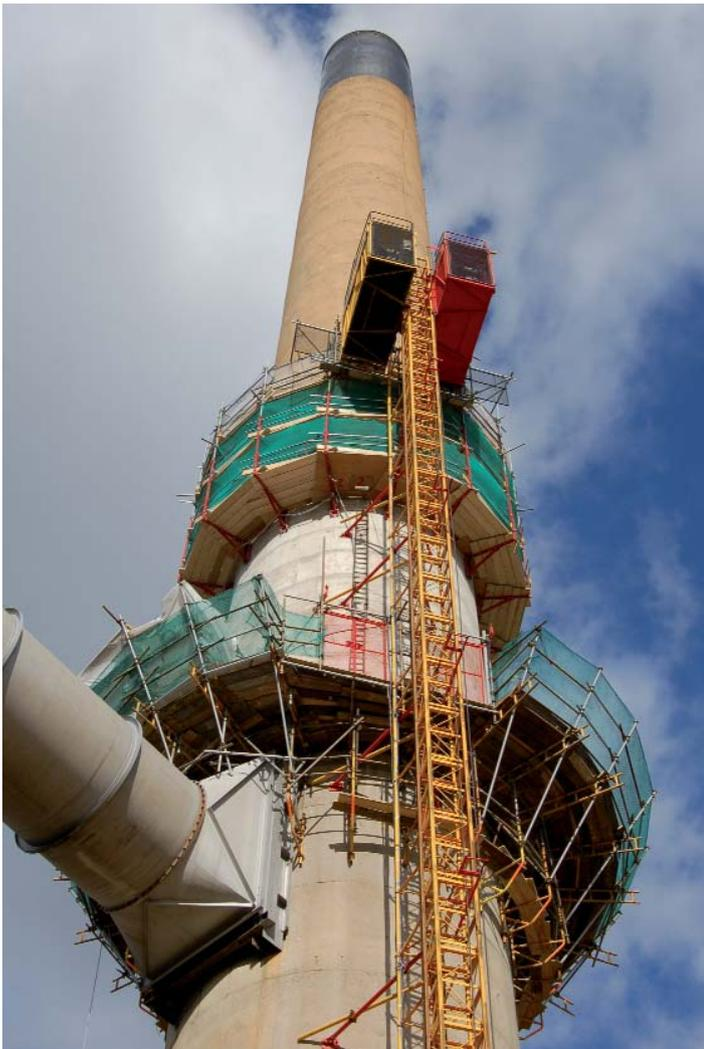
A radical new type of Climbing Platform powered by Control Techniques servo-drives controlling long reach actuators has been designed by Delta International, the UK's leading chimney contracting company.
