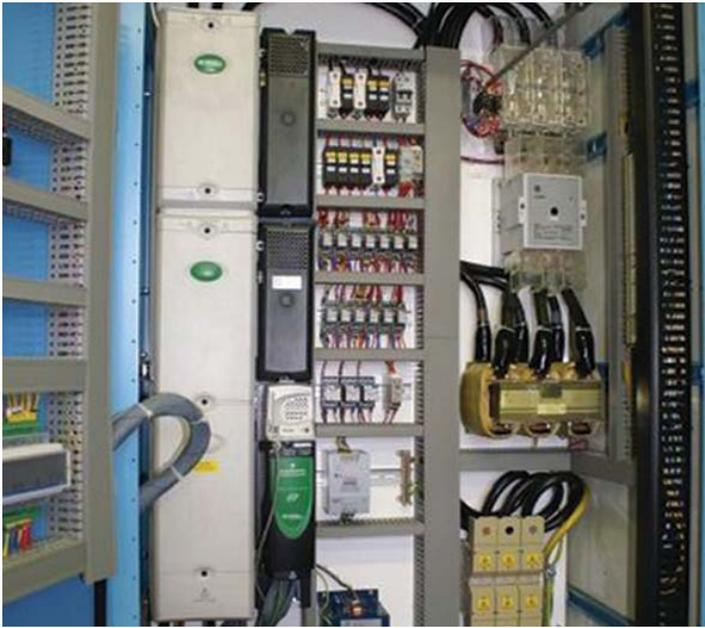
Applying Byzak's control philosophy in conjunction with Northumbrian Water's operational knowledge, the Project Team approached Control Techniques to develop a software package to satisfy the specification and to be suitable for running in the Unidrive SPs on-board PLC, the SM Applications module.
